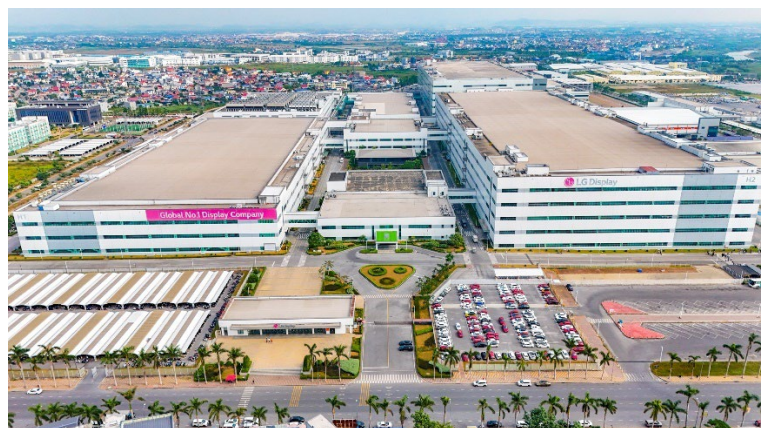
Figure 9: LG's Manufacturing Complex at Trang Due Industrial Park 1&2
